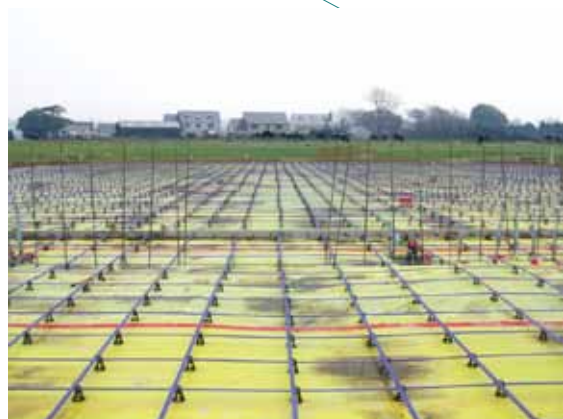
Slab on Grade
