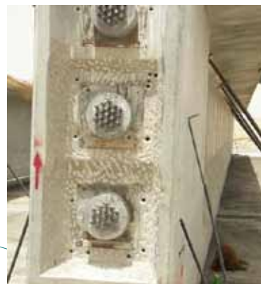
Installation of Anchors
