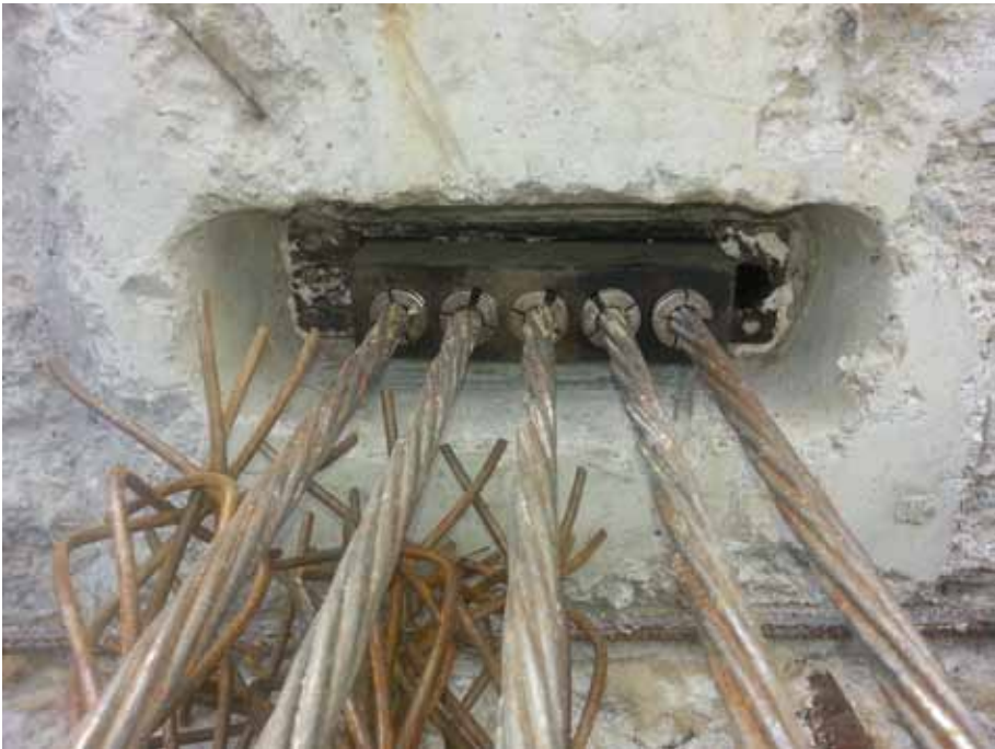
Installation of Flat Anchors
