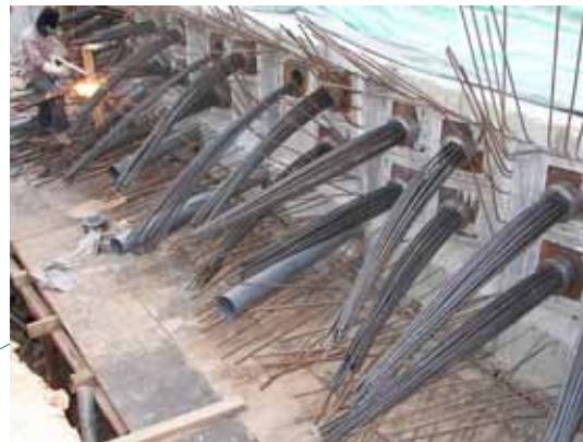
Installation of Anchors
