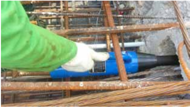
Stressing of Flat Anchors
