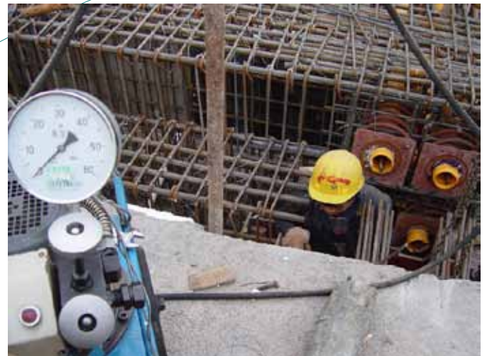
Preparation for Stressing
