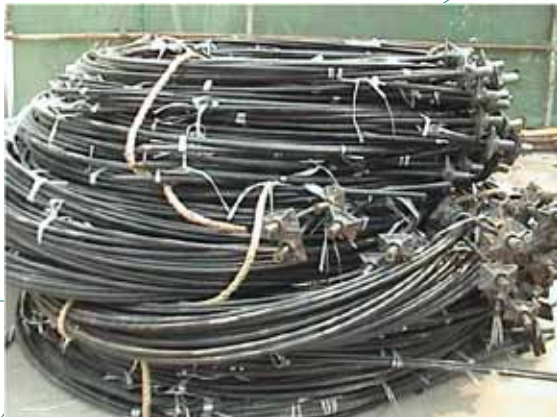
Prefabricated Unbonded Strands for Slab On Grade Application
