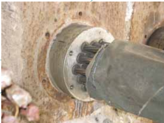
Installation of Anchors
