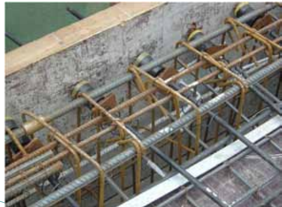
Slab on Grade
