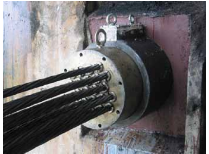
Installation of Anchors for Beam Stressing
