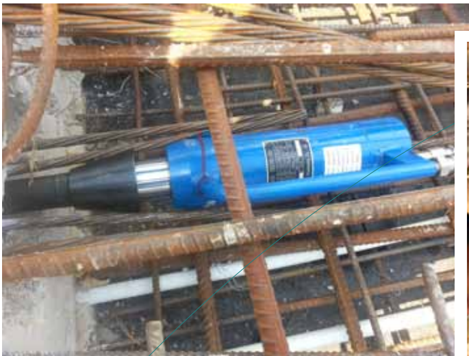
Mono Jack Stressing in Progress
