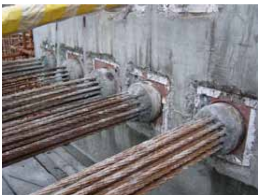
Installation of Anchors
