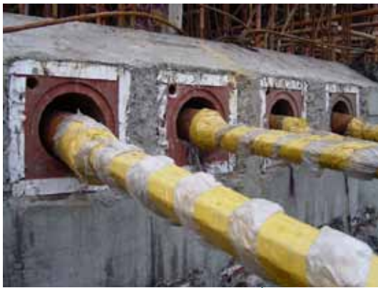
Installation of Anchors
