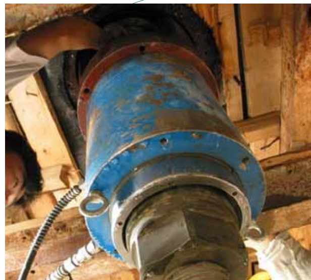
Installation of Stressing Jack
