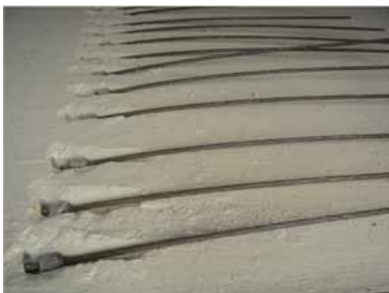
Slab on Grade
